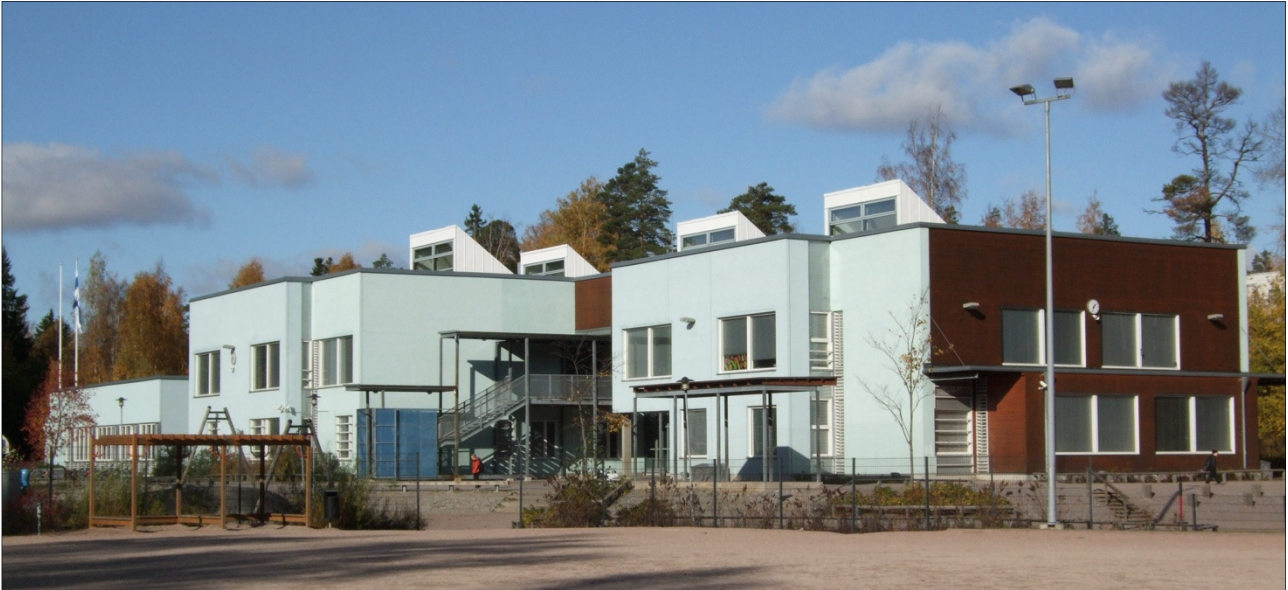
Figure 1. Front view of building.
