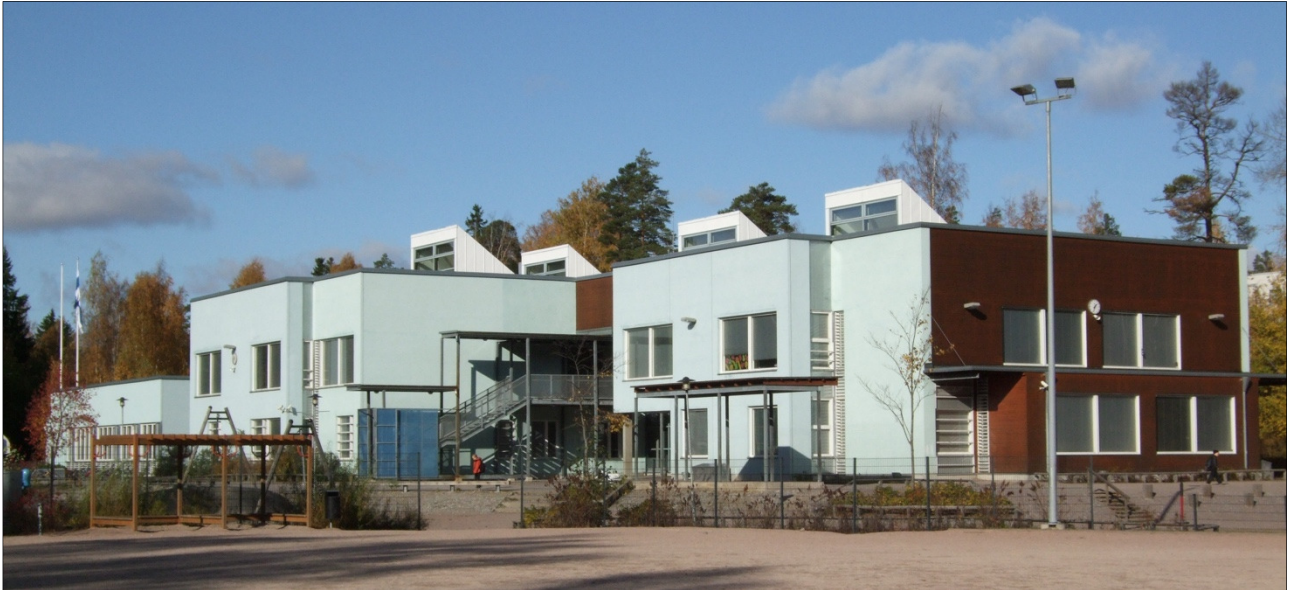
Figure 1. Front view of building.
